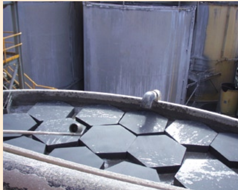
Resilient floating hexagonal barriers in place on a leach tank at Kalgoorlie Consolidated Gold Mines' operation in Kalgoorlie, WA during a trial by a Parker Centre team that showed that the barriers were effective in reducing diffusion of hydrogen cyanide gas ( \text{HCN}_{(g)} ) from the slurry surface. The trial was reported as part of the research on monitoring and minimising \text{HCN}_{(g)} emissions that was published in a paper in the May 2008 issue of the Minerals Engineering journal.
